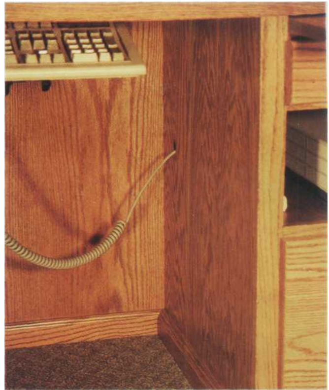
9 This detailed photo shows the hole cut in the drawer section's left bulkhead for the keyboard wire.
